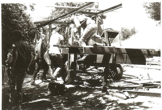
Now some wood-work - About April 1968
