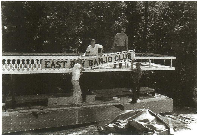
Almost finished May 1968
