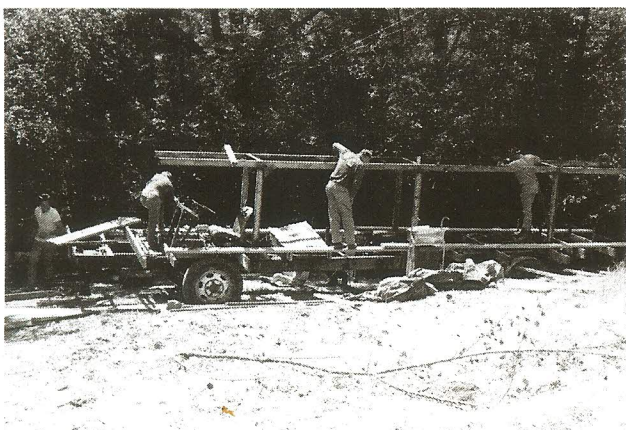
Building the float - The welders at work. Just starting March 1968
